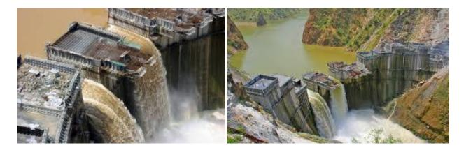
The above two pictures showed the Tekeze Hydropower dam. At the time of completion, the 188 meters (617 ft) high dam was Africa's largest arch dam. It was Ethiopia's largest public works project. The dam helped to reduce power shortages as Ethiopia's power demand increases.<sup>7</sup> The dam is functional and generating power from Tekeze River.
